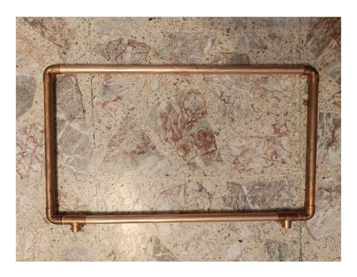
Once you have all angles and "T" connections glued, press all sides firmly against a flat hard surface, and leave it overnight to complete curing. Its important that all edges and sides are touching the floor so everything is perfectly flat, make sure all tubes fully inside.
